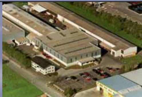
WAG Büren Production facility with ultra-modern sheet metal processing facility.
